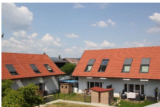
© David Bliemegger (nachher)
